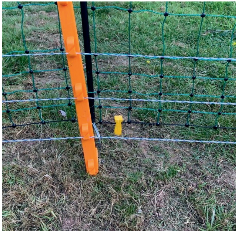
Figure 8: Electric Rabbit Fencing & Figure 9: Inner 3 row fencing & outer rabbit fencing with pegs to secure © Shropshire Badger Group
