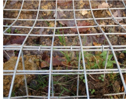
Figure 21. Hog rings connecting fencing.
